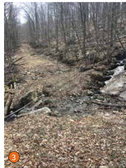
3 There are 13 culvert washouts on the access road.
