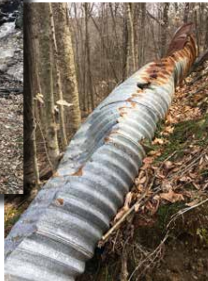
3 There are 13 culvert washouts on the access road.
