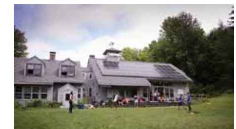
Roof-mounted solar at Tamarack Farm.
