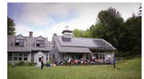
Roof-mounted solar at Tamarack Farm.
